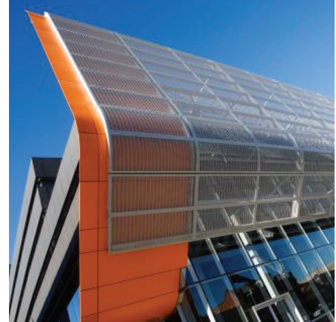
* Typical architectural installation.
